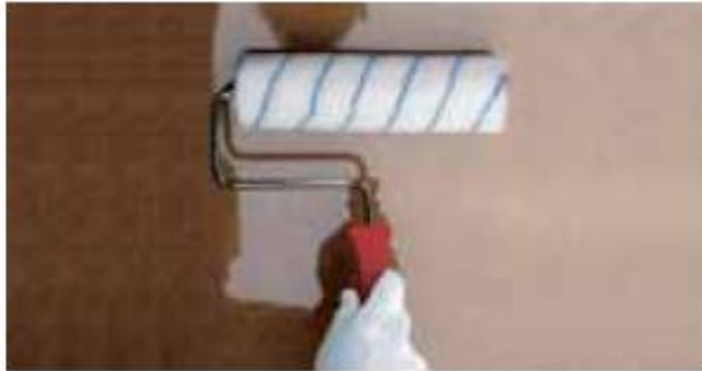
Primer application with medium long pile roller
