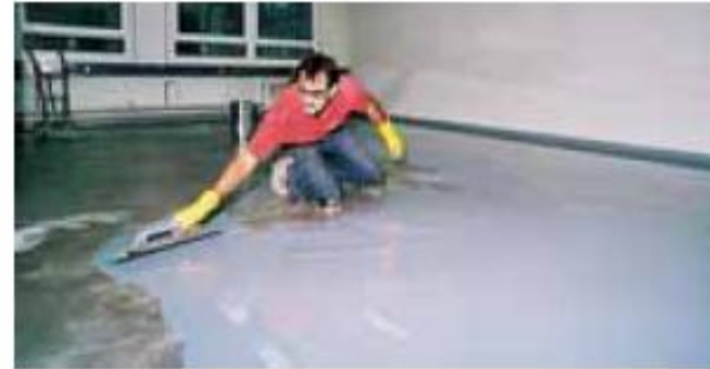
Application of a self smoothing screed with a notched trowel
