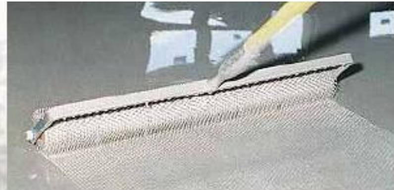
Spiked rolling immediately removes any entrapped air
