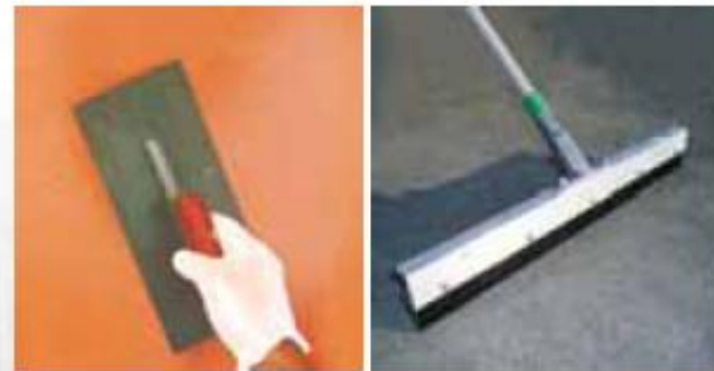
Sealing of a broadcast layer with a straight trowel or "squeegee" blade
