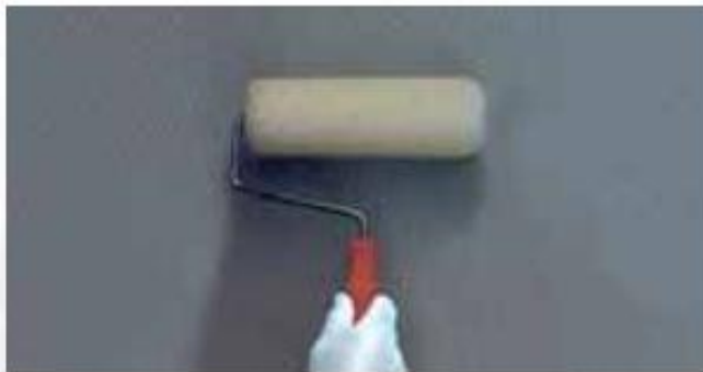
Application e.g. of Sikafloor®-261 Thixo with a textured roller
