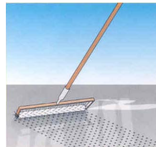
Removal of entrapped air: Spike rolling immediately e.g. Polyplan spike roller.
