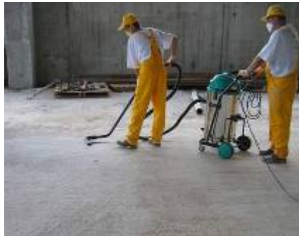
Cleaning of the surface
