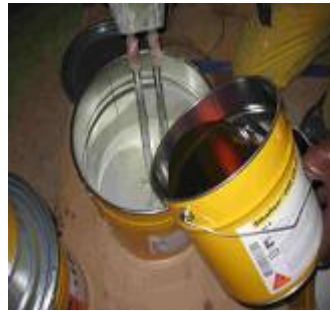
Mixing of Sikafloor®-169
