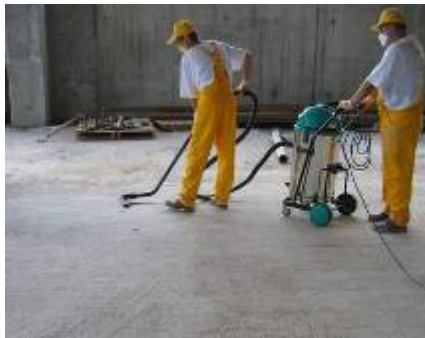
Cleaning of the surface
