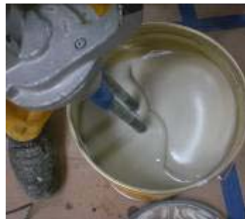
Mixing of Sikafloor®-169 and Sika® -Compact Filler
