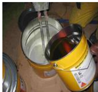
Mixing of Sikafloor®-169
