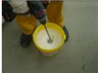
Mixing of Sikafloor®-304 W
