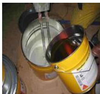
Mixing of Sikafloor®-169
