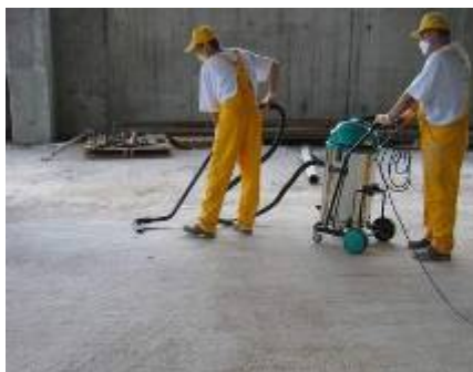
Cleaning of the surface
