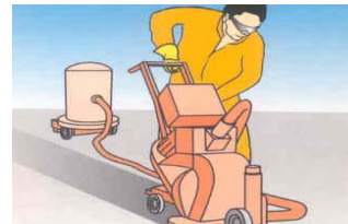
Preparation of the substrate: Blast cleaning or other mechanical means. E.g. Blastrac.
