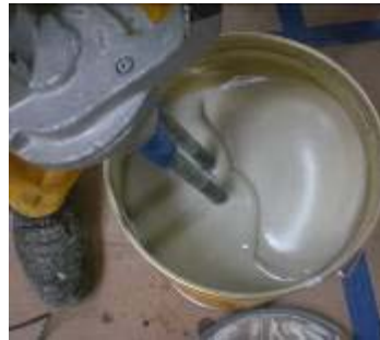
Mixing of Sikafloor®-169 and Sika® -Compact Filler
