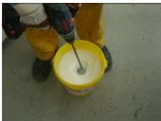
Mixing of Sikafloor®-304 W
