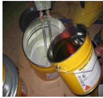
Mixing of Sikafloor®-169
